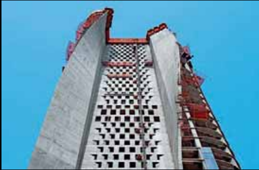
This page: Building under construction Opposite: Daytime view
