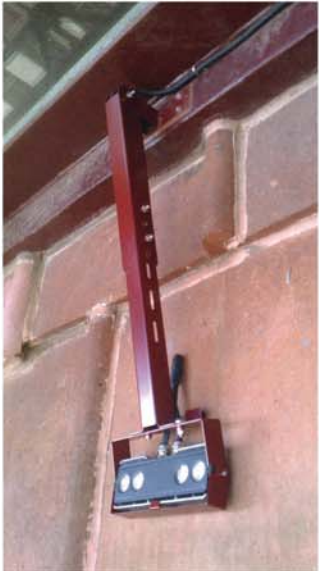
View of facade ledges from inside the Rookery Building. Luminaire positions had to work around the intermittent ribbed detailing at all of the ledges.
